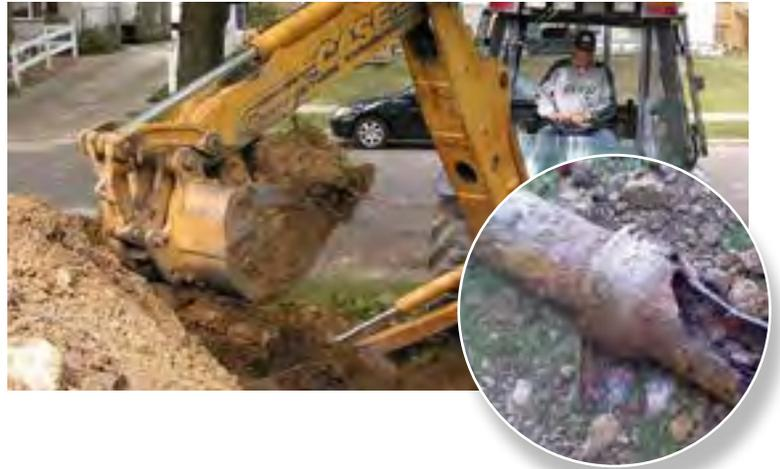
Last Christmas season, David was shocked to learn that an old clay sewer pipe deteriorated in his front yard, and he was responsible for its repair. That meant digging up his driveway. It cost him \$3,500 to replace the sewer pipe with PVC piping and another \$4,000 to excavate and repair the driveway.
